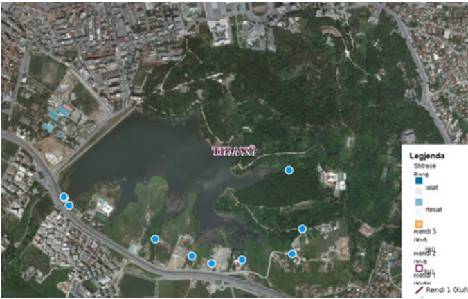
Key field findings from the Environmental Audit on the Artificial Lake of Tirana
