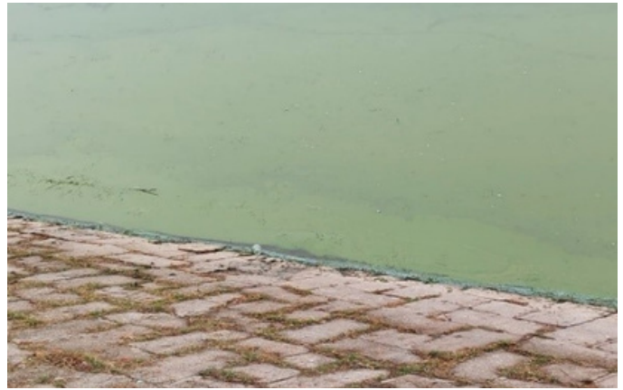
Photos from the on-site verification conducted by the audit team.
